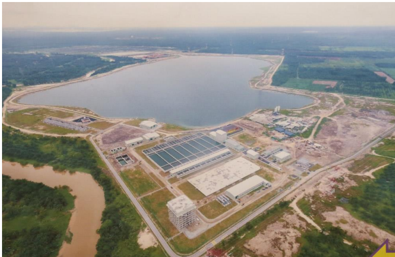
LRA Labohan Dagang – Maintenance Work
